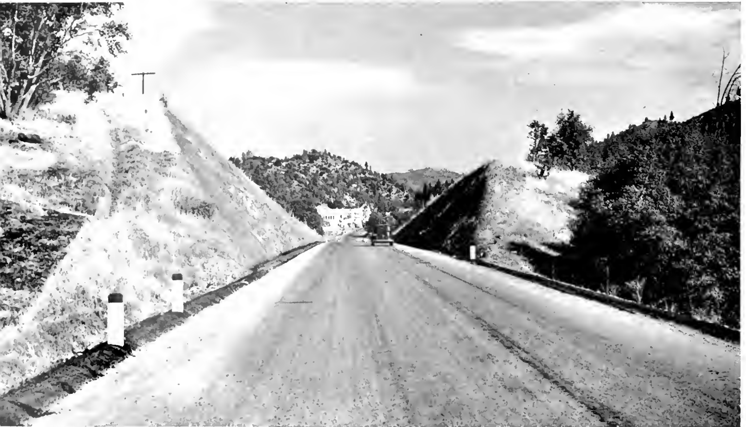
New All-Year Yosemite Highway relocation goes straight through Mariposa obviating right hand turns of old route on city streets
